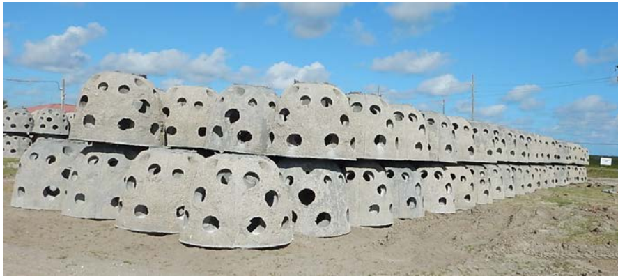
Artificial reef domes just before they were placed in the northern nearshore waters in April 2017.
