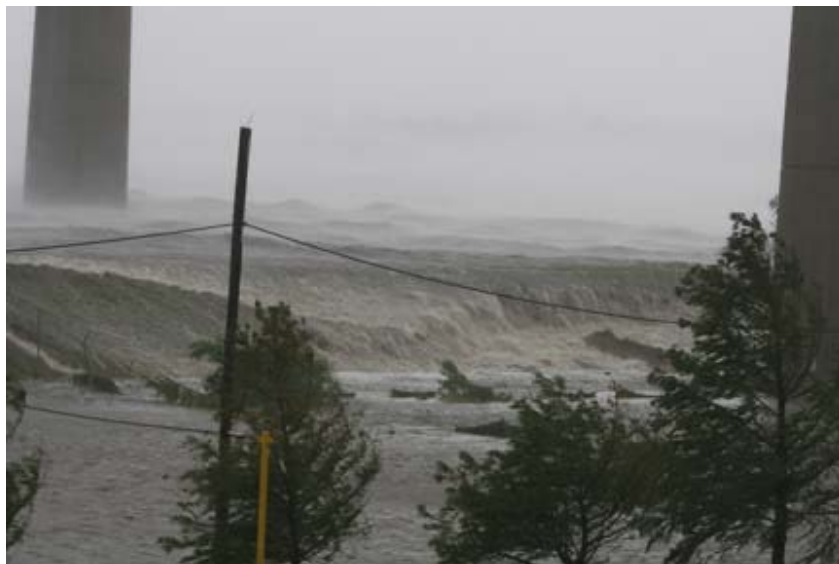
Photo taken by Don McClosky from the Entergy Michoud Plant located beneath the I-510 bridge over the GIWW (note the concrete piers of the bridge in the photo). Water is cascading over the 17 ft levees, and note the wave of water above the levee that is moving left to right (east to west) in the photo.
