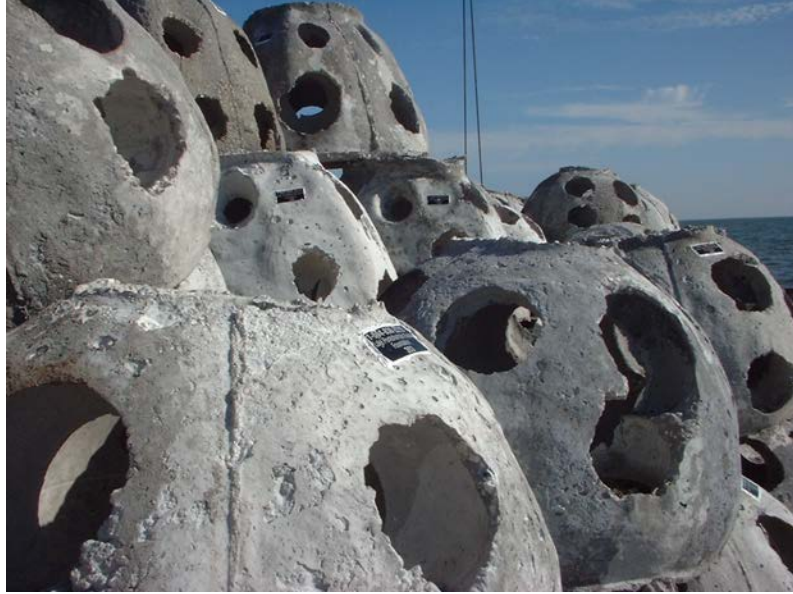
Artificial reefs about to be placed on the lake bottom. Courtesy the Lake Pontchartrain Basin Foundation.
