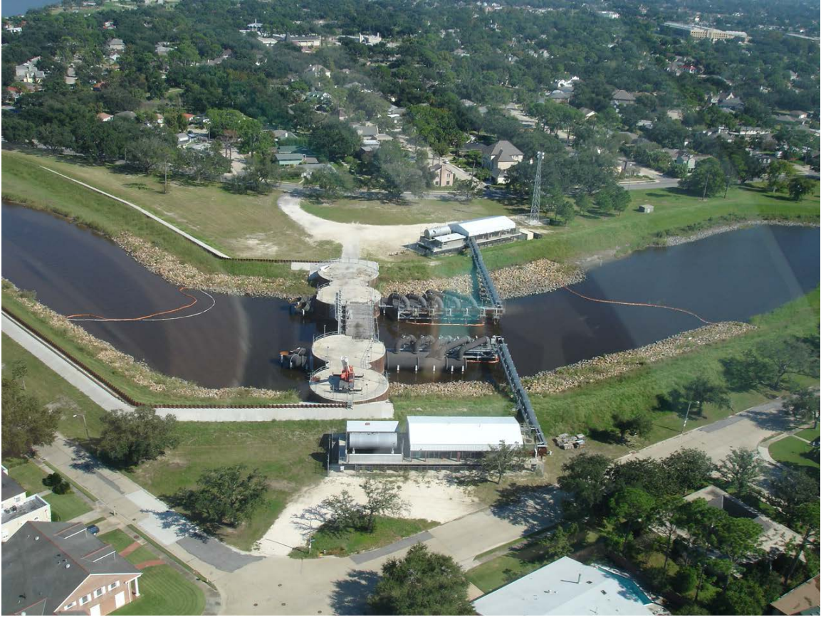
In order to prevent future surges from the lake repeating the Katrina disaster, each of the levees has floodgates that are closed when a storm enters the Gulf of Mexico. The gates have pumps that allow floodwater resulting from rains to be pumped into the lake against the head of water that may exist. This photo is of the floodgates on the Orleans Canal.
