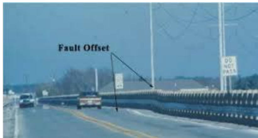
A "fault offset" is visible on the south bound lanes 3.1 miles from the toll booths. The image above was taken when there were only 2 lanes on the Causeway. Source: Environmental Atlas of Lake Pontchartrain.
